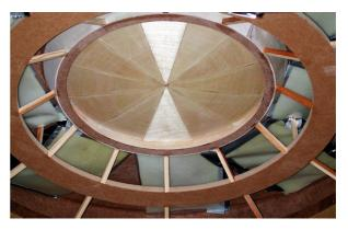
**Figure 18.** Membrane absorbers inserted in the roof of the auditorium.
