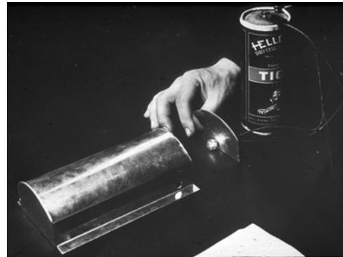
Fig. 3. Optical model of a hall with a concave ceiling. The energy distribution on the floor can be studied on a photographic plate.
