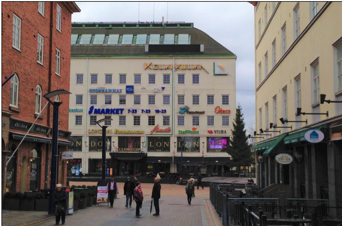
Figure 1: The Kolmikulma shopping center, showing the rehearsal hall roof windows in the attic.
