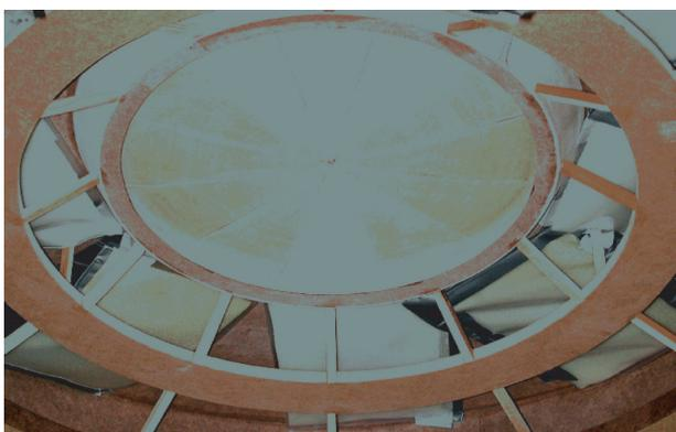
Figure 18. Membrane absorbers inserted in the roof of the auditorium.
